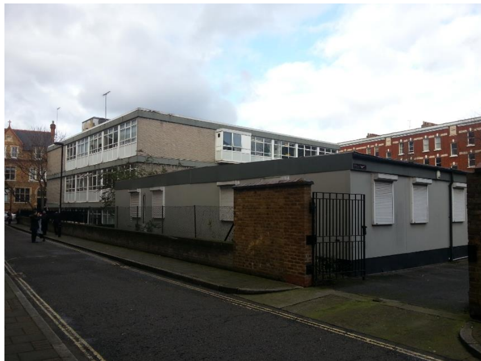
View of Shroton Street elevation (top) and view north along Stalbridge Street (bottom).
