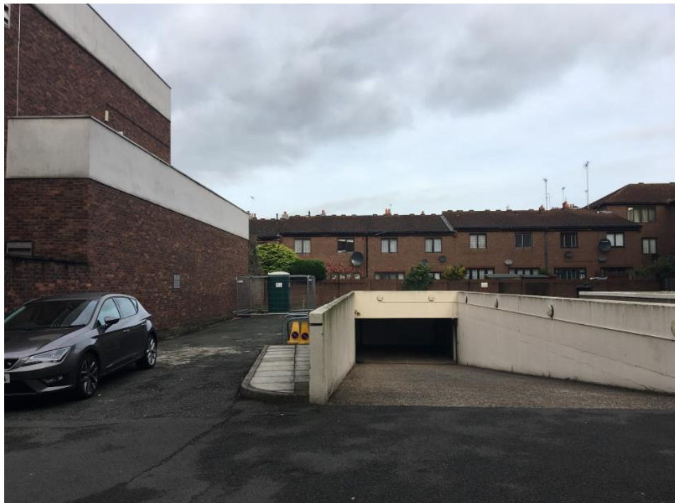
Views of existing landscaping to area between the Repeater Station, Alpha House and Earl House including existing vehicular ramp.
